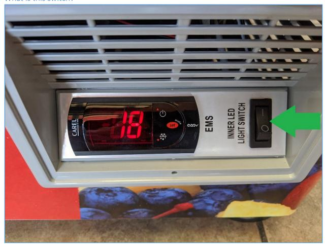
This switch turns the internal **light** on/off. It does **NOT** turn the machine on/off!
